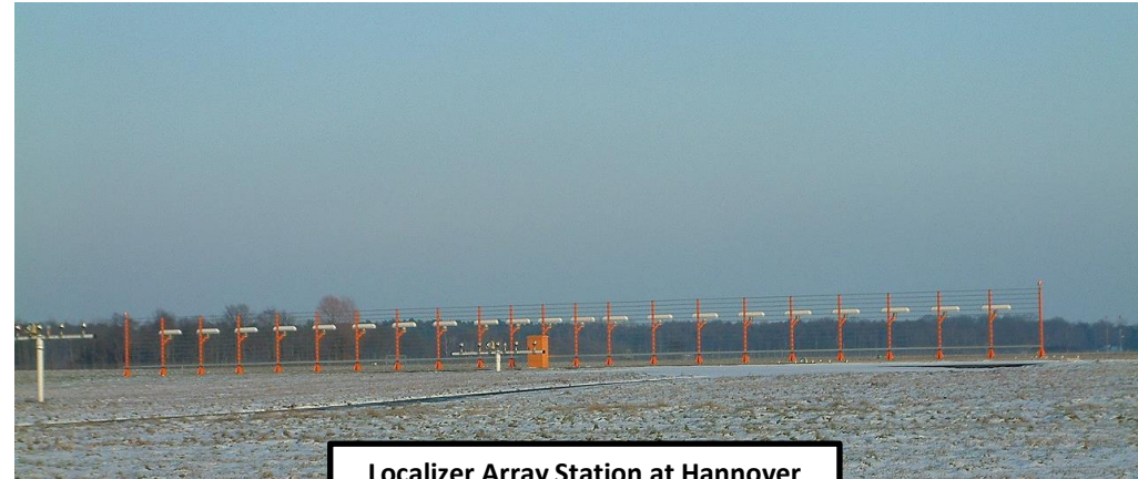
Localizer Array Station at Hannover
